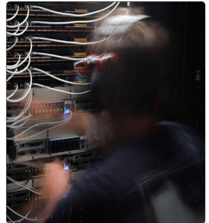
Increasing Infrastructure Complexity Requires Rich Ecosystem and Common Infrastructure
